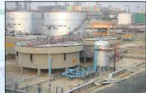
Dissolved Air Flotation
