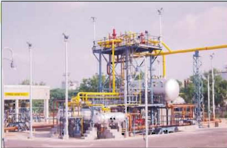
EPC Execution of Gas Gathering Station for ONGC
