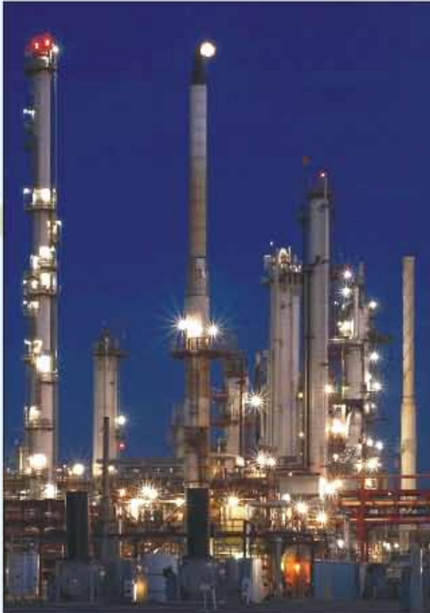
Commissioning Assistance at Bharat Oman Refineries Limited
