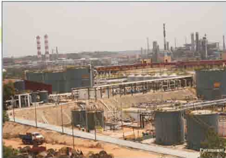
One of India's Largest Industrial Waste Water Treatment & Recycle Plant at M/s. Mangalore Refinery & Petrochemicals Ltd. (Phase III Refinery Project).
