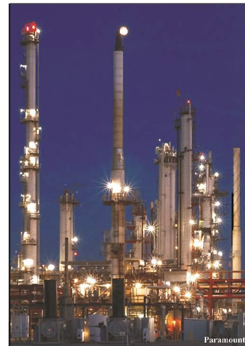
Commissioning Assistance at Bharat Oman Refineries Limited
