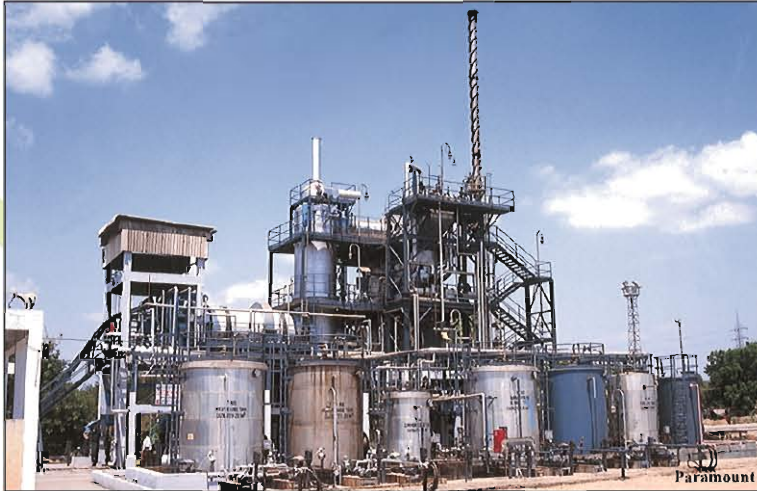
2000 T/Yr Incinerator at Reliance Industries Ltd., IPCL, Baroda
