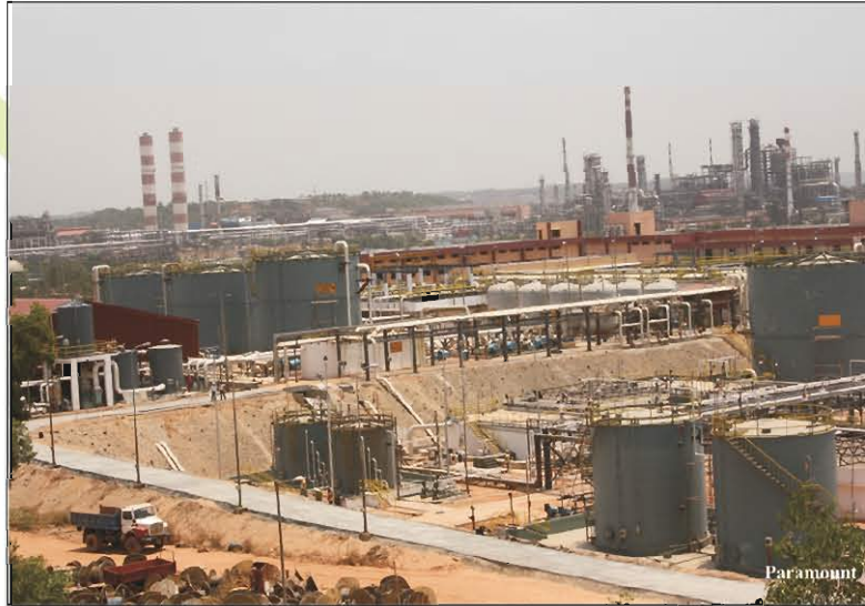
One of India's Largest Industrial Waste Water Treatment & Recycle Plant at M/s. Mangalore Refinery & Petrochemicals Ltd. (Phase III Refinery Project).
