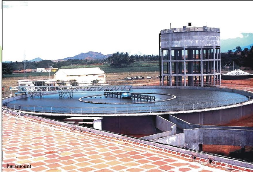
RWTP with overhead tank at Madurai
