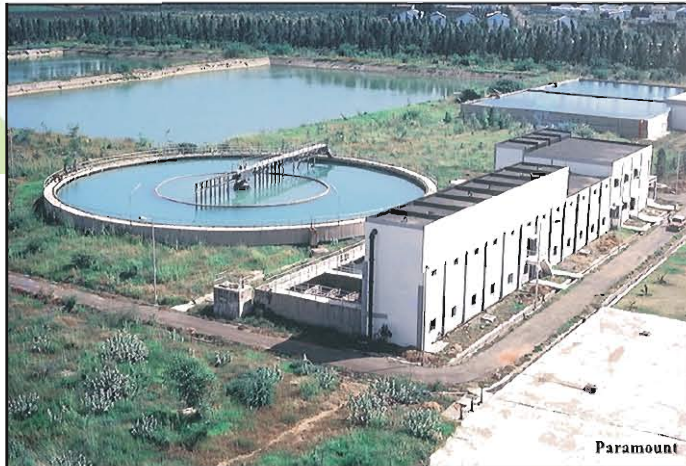
Raw Water Treatment Plant at GNFC, Bharuch
