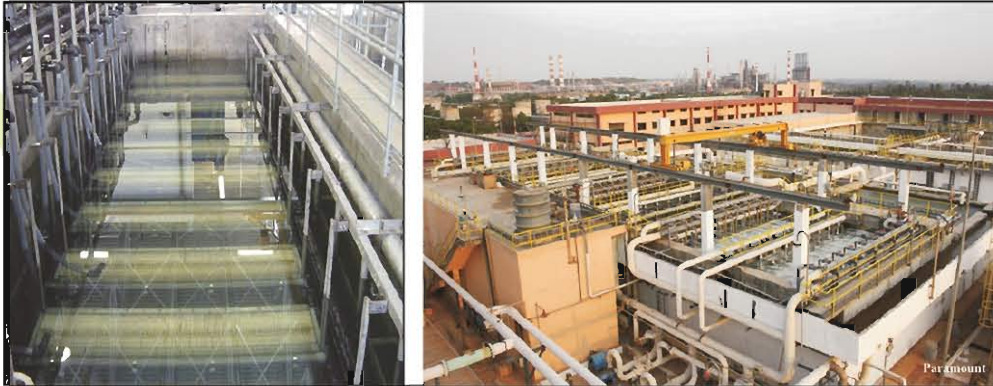
Flat Sheet Membrane Mangalore Refinery & Petrochemicals Ltd., Mangalore (MRPL)
