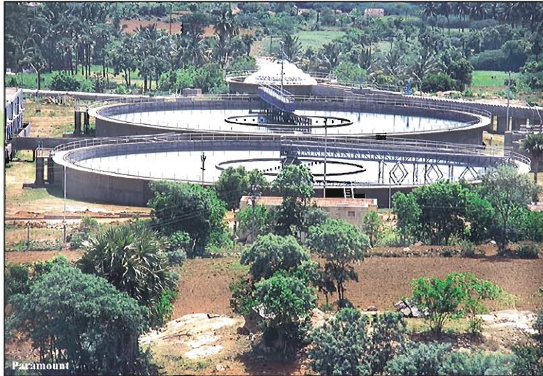
RWTP with overhead tank at Salem
