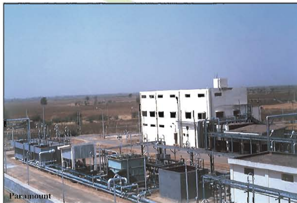
Water Re-injection Plant & ETP for ONGC, Mehsana
