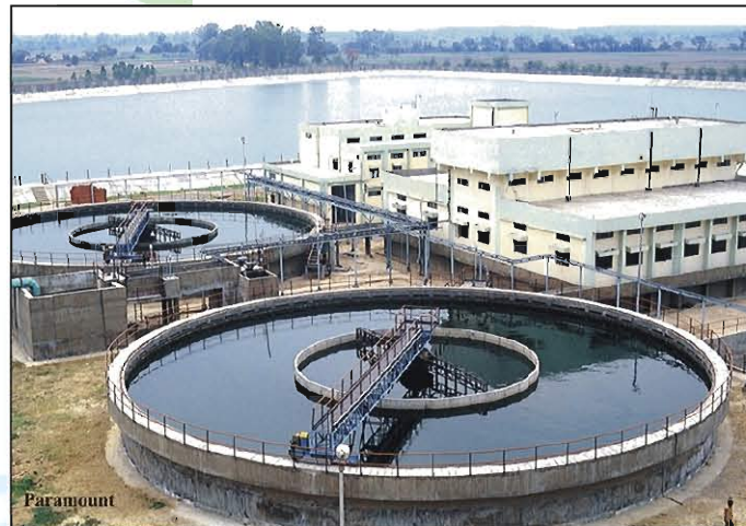
110 MLD Intake Channel, RW Reservoir & WTP for ONGC
