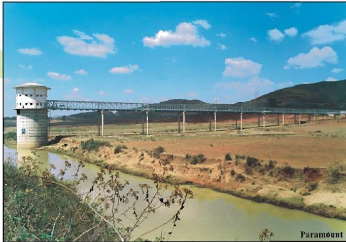
Intake Well at NALCO
