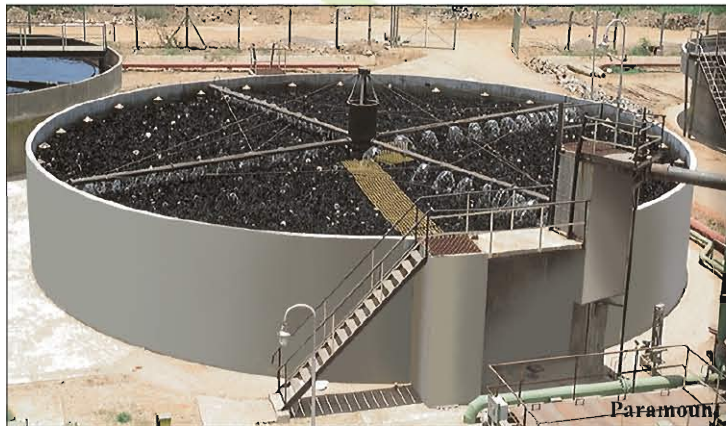
Plastic Media Bio-Tower Alembic Limited, Gujarat
