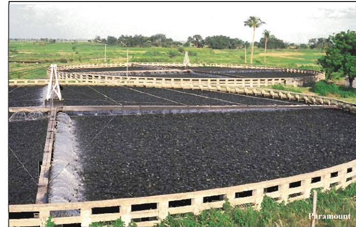
28 MLD STP at Wadi for Municipal Sewage & Industrial Effluents
