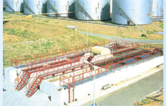
TPI for a oil tank farm
