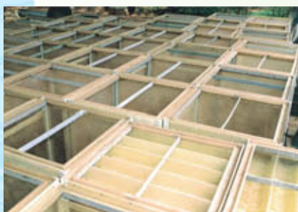
Plate packs under assembly
