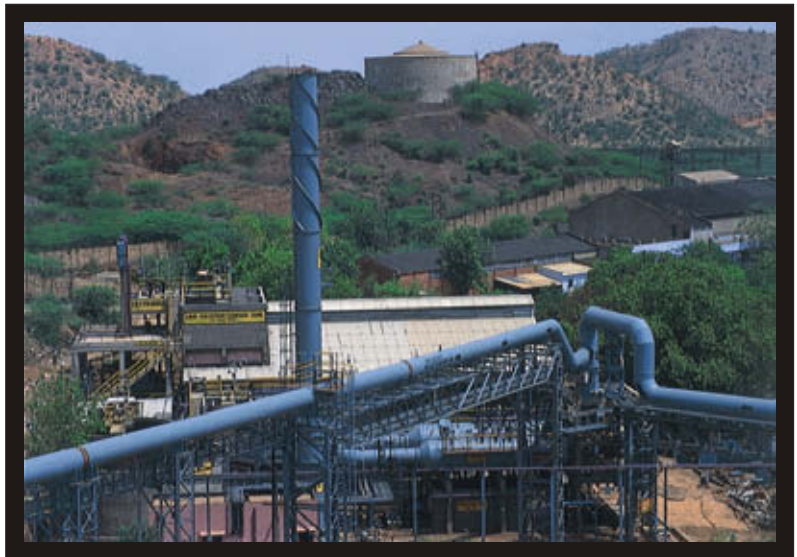
FGD with Double Alkali Process at a Copper Smelter
