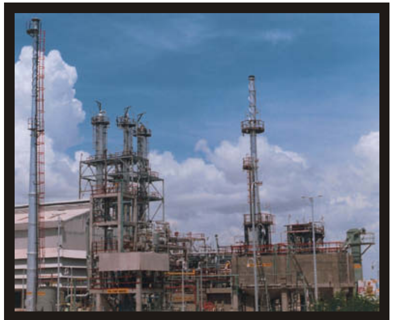
Acid Gas Incinerator with Double Alkali Process
