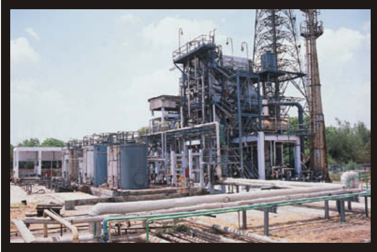
Rotary Kiln Incinerator plant with Particulate/ \text{SO}_2 /HCl Scrubbers
