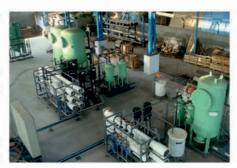
Skid mounted CIP (chemical in plant) units are the norms of PARAMOUNT design to enable effective periodic cleaning of RO membranes.
