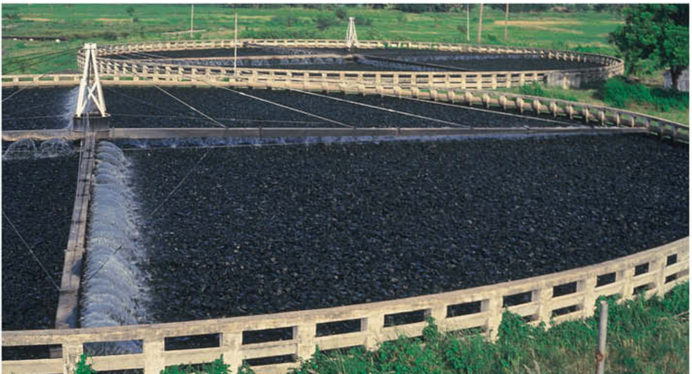
..... Trickling filter for a Municipal Sewage treatment
