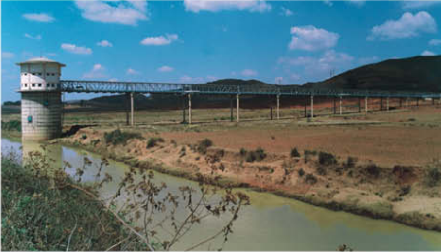
Intake structure at a river bed
