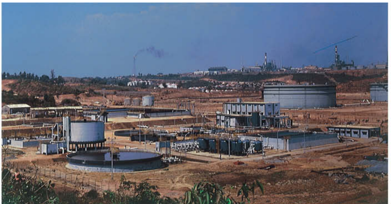
Bird's eye-view - Effluent treatment plant at a 6 MMTPA Refinery
