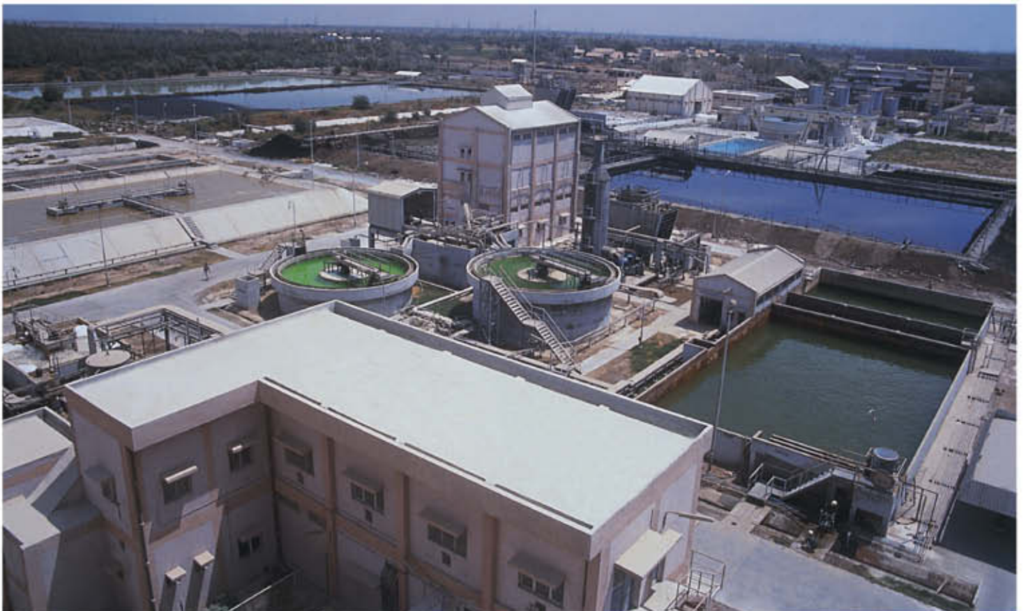
Effluent treatment plant for removal of phosphates, fluorides & nitrates at a Nitrophosphate fertilizer plant
