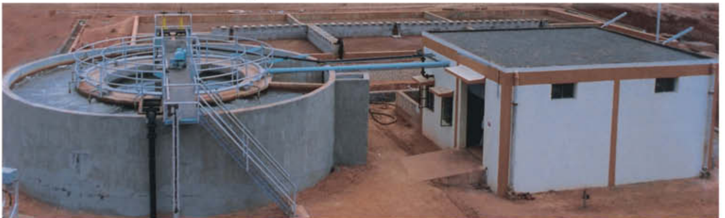
Package sewage plant for a colony .....
