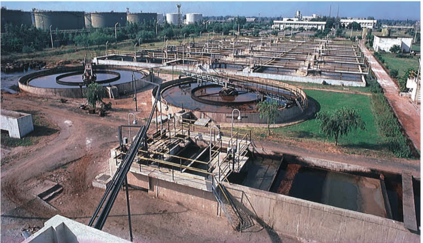
Central effluent treatment plant at an integrated Petrochemical complex
