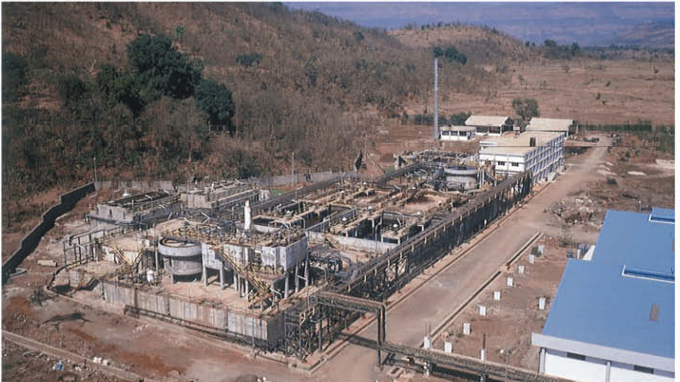
Bird's eye view of an integrated four stage (primary, anaerobic, aerobic and tertiary) treatment facility for a pharmaceutical unit
