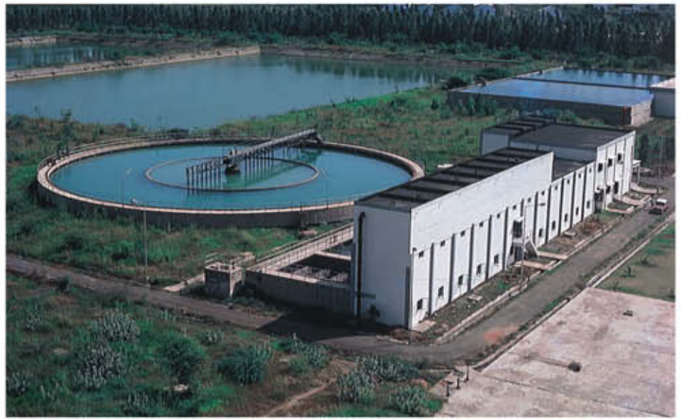
Water treatment plant at a Fertilizers complex
