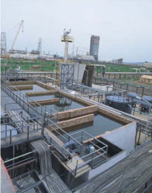
Chromate removal facility for Cooling tower blow down at a Fertilizer Complex
