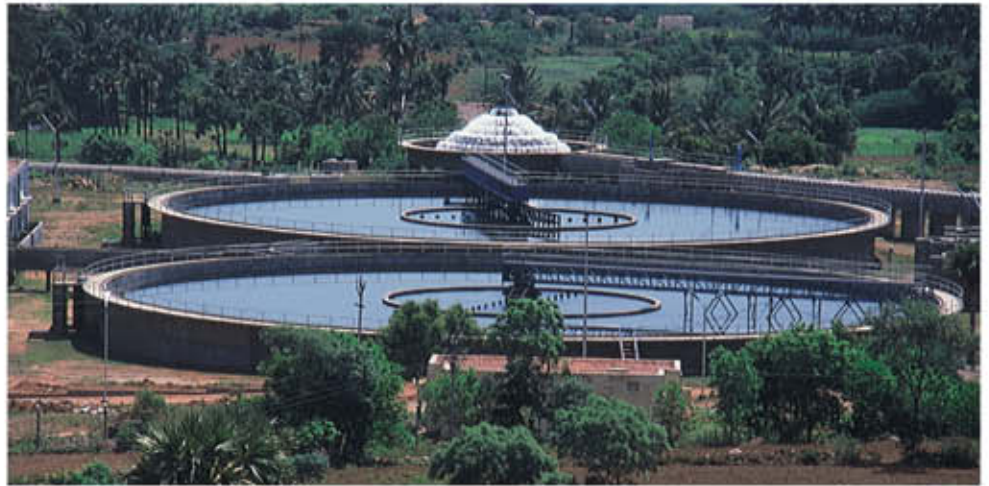
Water treatment plant for a large community
