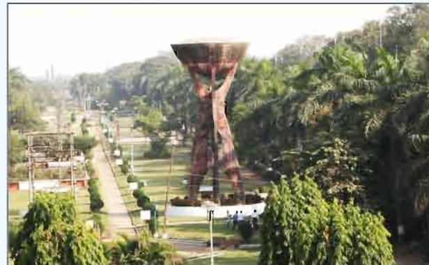
Lalbag OverHead Tank, Vadodara
